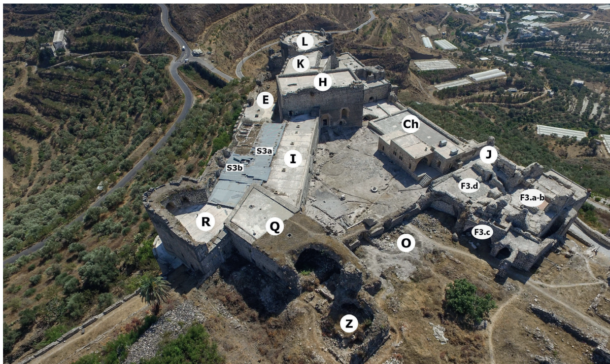
• Fig. 5. Aerial picture of the castle from the north with the code of the main buildings indicated. By B. Takáts
