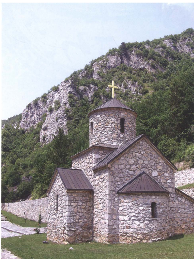
Fig. 6. Monastery church after restoration
