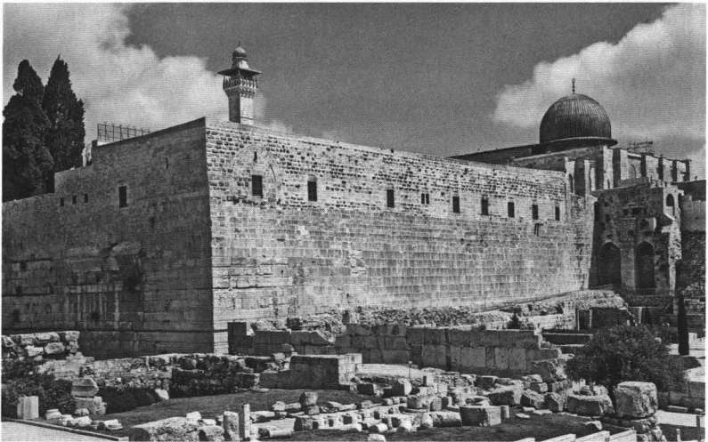
Fig. 23. The southwestern corner of the Temple Mount (photo by G. Laron). Note the original Herodian lower courses and smaller stones of a later reconstruction above
